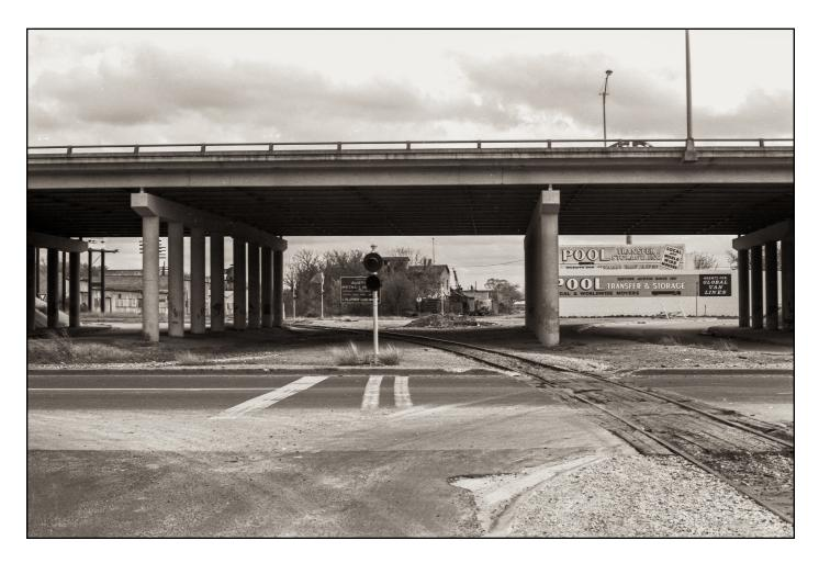
Forth Street at IH35 facing east. The crossing signal's upper head flashed and the lower head displayed "No Right Turn."
