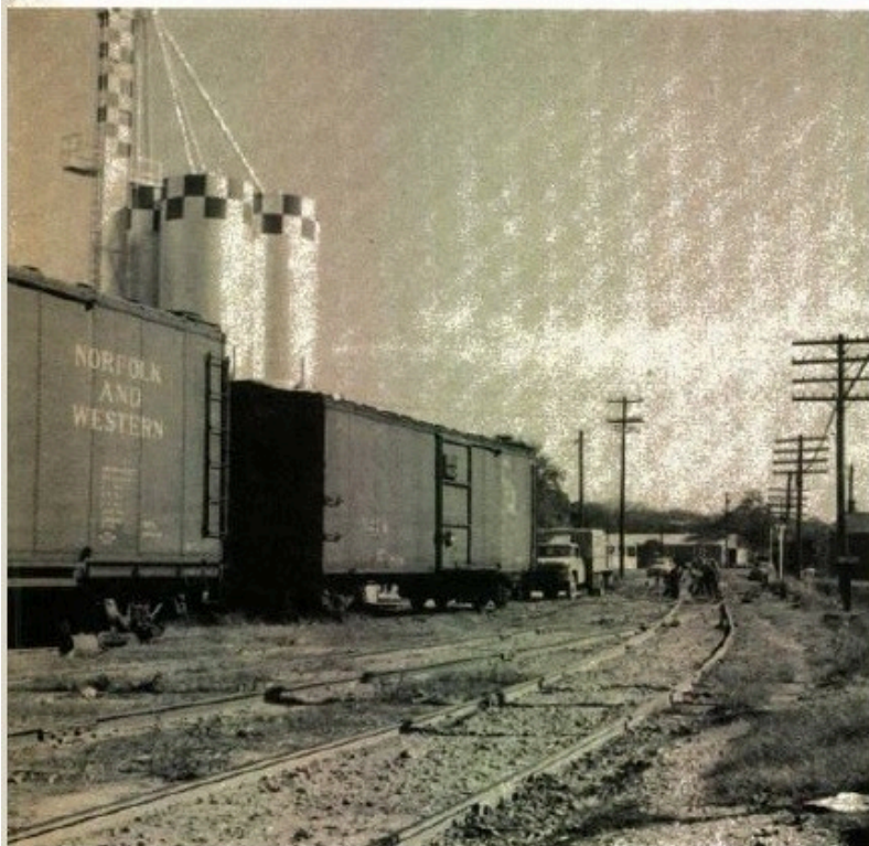
Main line where it has just left street is so covered with gravel and dirt you cannot see the ties. In modeling, note how soil rises to each side of track. This continues a little way until track can reach a better-drained level. Note also path worn through weeds, parallel to track.
